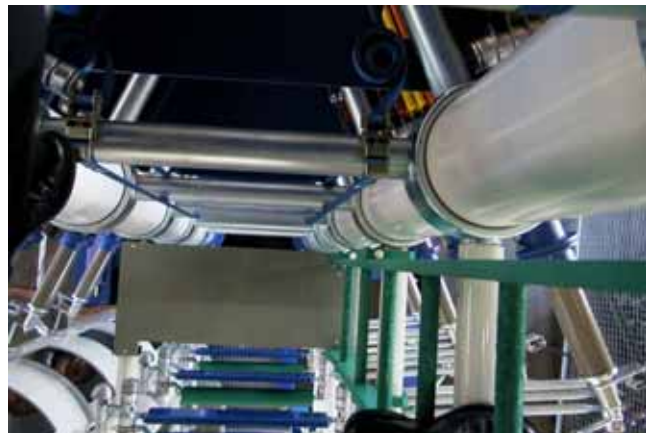
Internal view of ladder and platform
