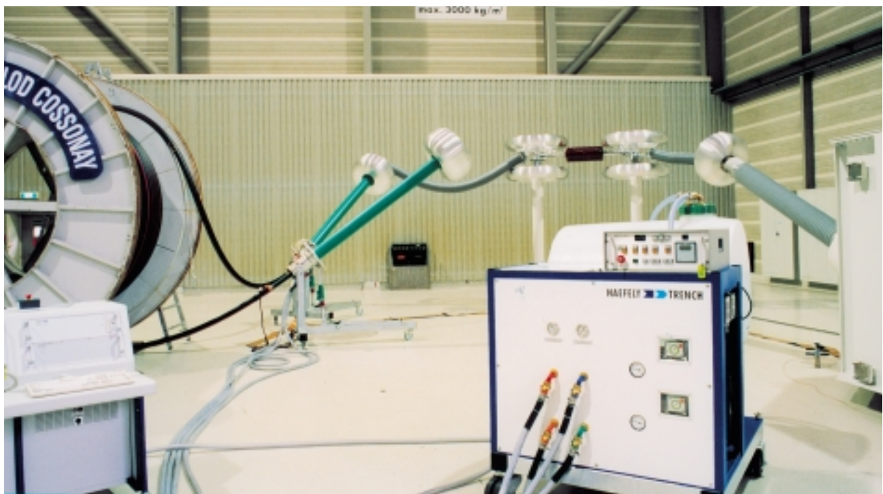
110 kV power cable under test conditions
